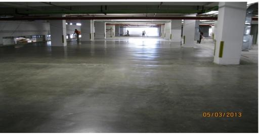
GREEN-POLISHED CONCRETE is an environmentaly friendly system that combines of "green" concrete blinder likes recycled glass. The densifier produces a substantially denser concrete surface with enhanced durability.
